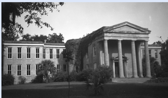
Historic photo of the Beaufort College Building with addition.
