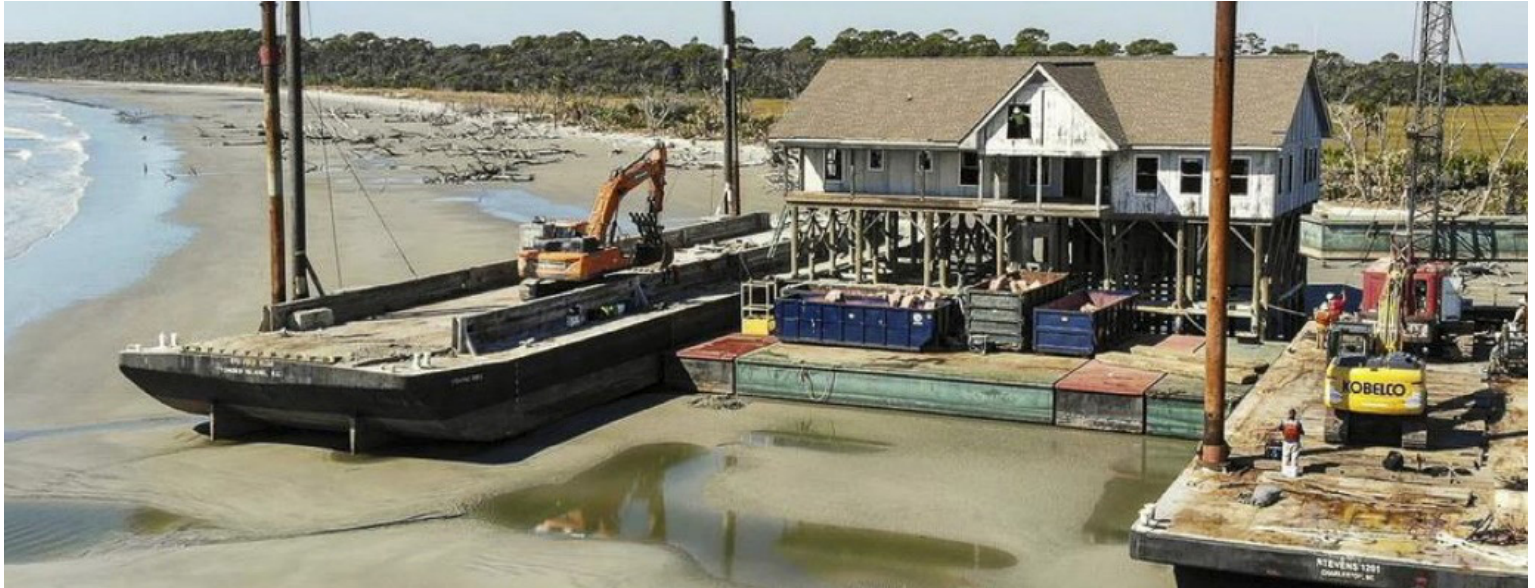
Beginning preparations for the lab building removal and clean up.
